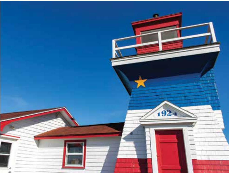
Salmon River Lighthouse in West Pubnico | All photos: Municipality of the District of Argyle
