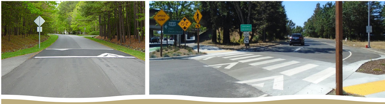
Figure 7: Examples of Traffic Calming. L: Speed table on a Rural Road, R: Raised crosswalk. (Photo credit: Small Town and Rural Design Guide)
