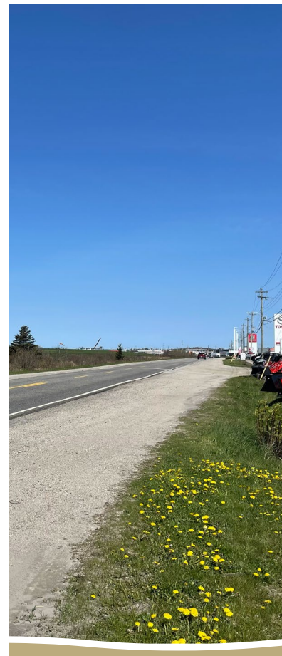
Figure 38: Airport Stretch Existing Conditions
