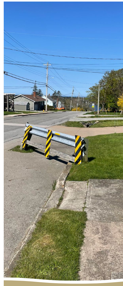
Figure 51: Prospect Street Crossing Existing Conditions
