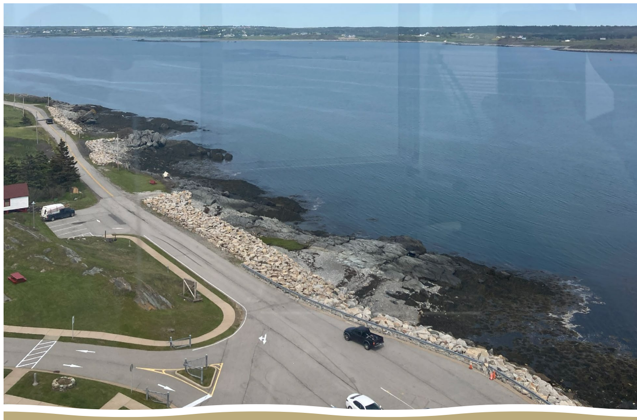
Figure 39: Cape Forchu Existing Conditions
