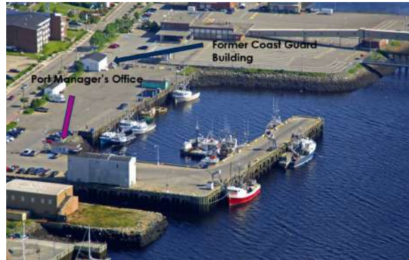
Former Coast Guard building.
